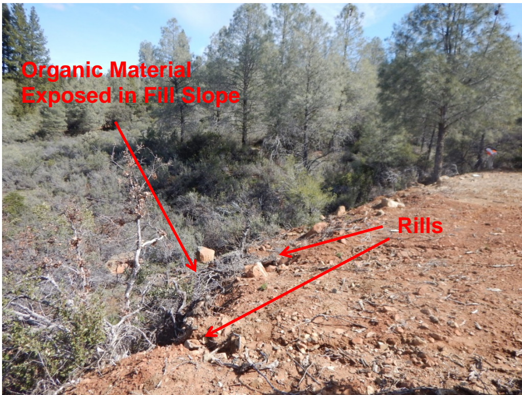
Photograph 5: Rills & organic material in lower fill slope. Photo by Kason Grady.
