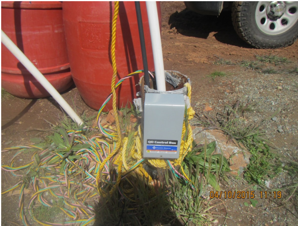
Photograph 12: Uncapped water supply well at location W1. Photo by Erin Mustain
